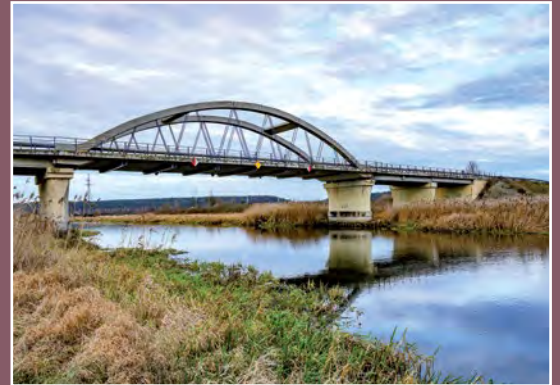
Most na Noteci Netzebrücke
