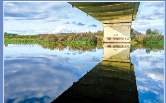
Most na Noteci Netzebrücke
